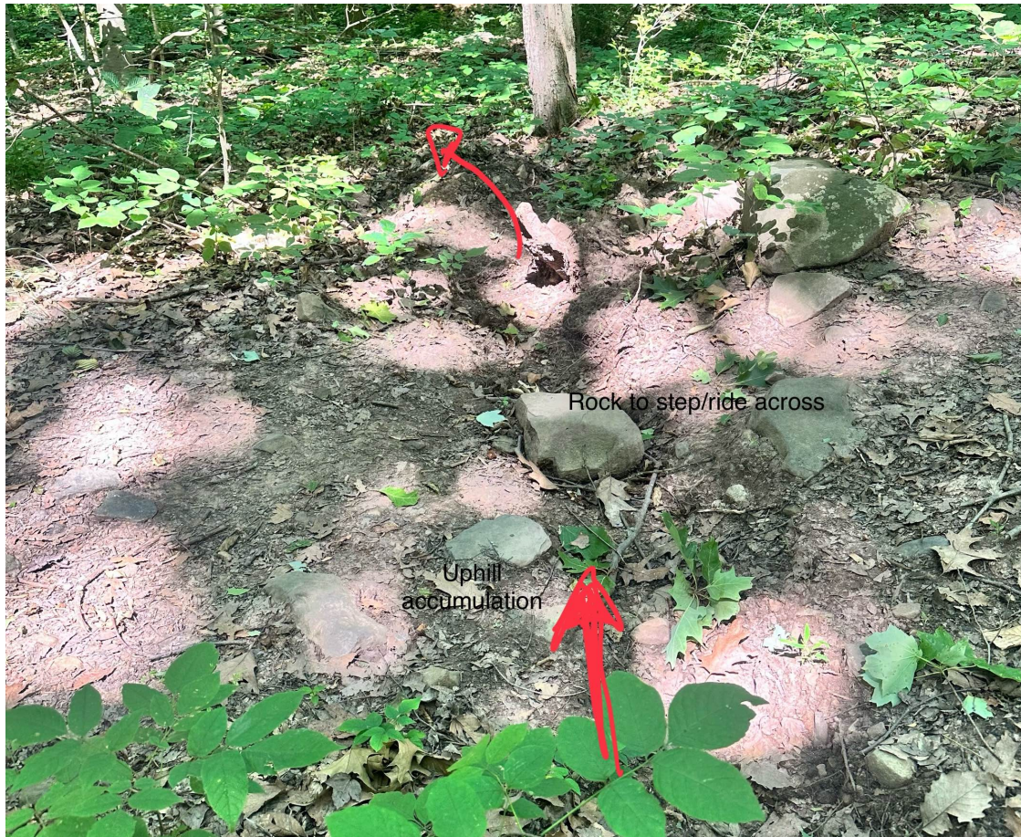
Figure 3.3: Example ford dug so deep a rock is placed to step/ride across
