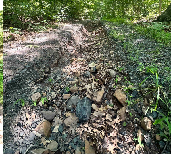
(b) Massive erosion on Hillspur trail
